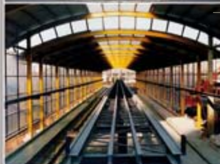
■ CFF railway carriage washing center (Switzerland) Design and project management
