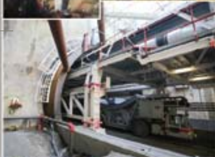
■ Mont Sion tunnel on A41N highway (France) Advisory services to client
