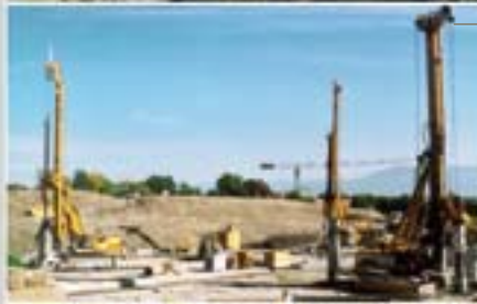
■ Tuileries water treatment facility (Switzerland) Geotechnical studies Design and project management
