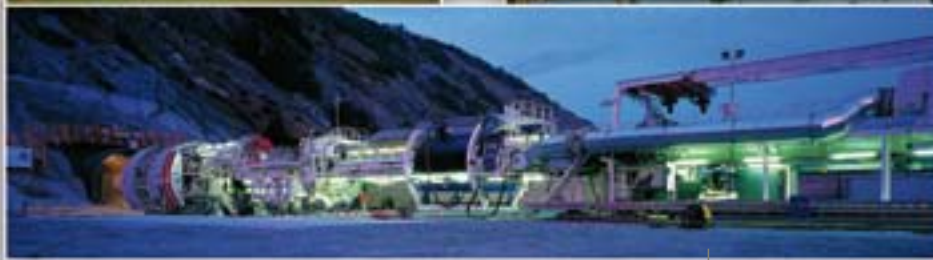
■ Lötschberg railway tunnel (Switzerland) Design and project management
