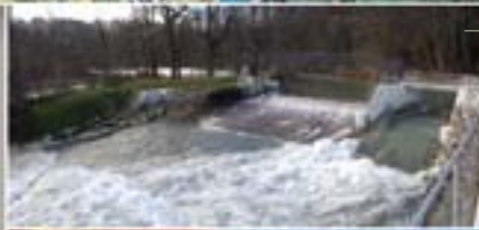
■ Vessy dam on the Arve River (Switzerland) Design and project management
