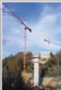
■ Usses Viaduct on A41N highway (France) Advisory services to client
