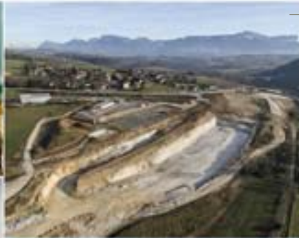
■ Noiret cut-and-cover tunnel on A41N highway (France) Advisory services to client
