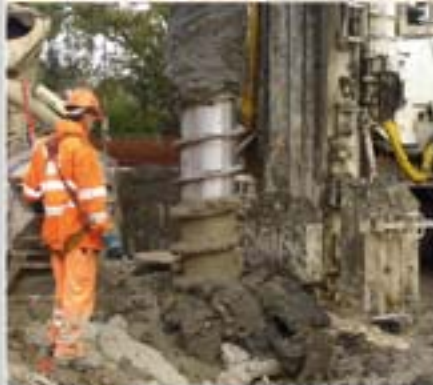
■ Bored piles with a hollow auger
