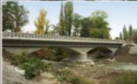
■ Allondon bridge rehabilitation (Switzerland) Design and project management
