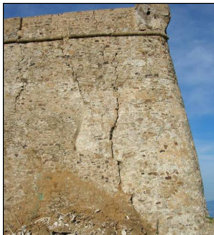
Figure.12. Ensemble de fissures des fortifications Sud. Cracks of the south fortifications.
